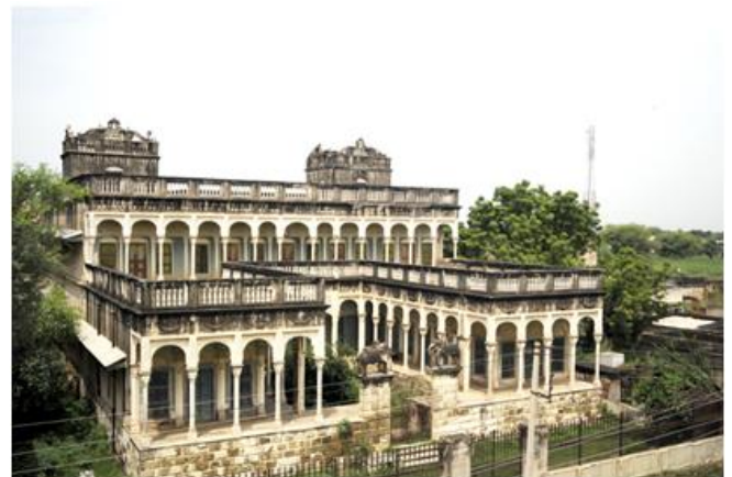
Fig 7: Haveli of Rajasthan
